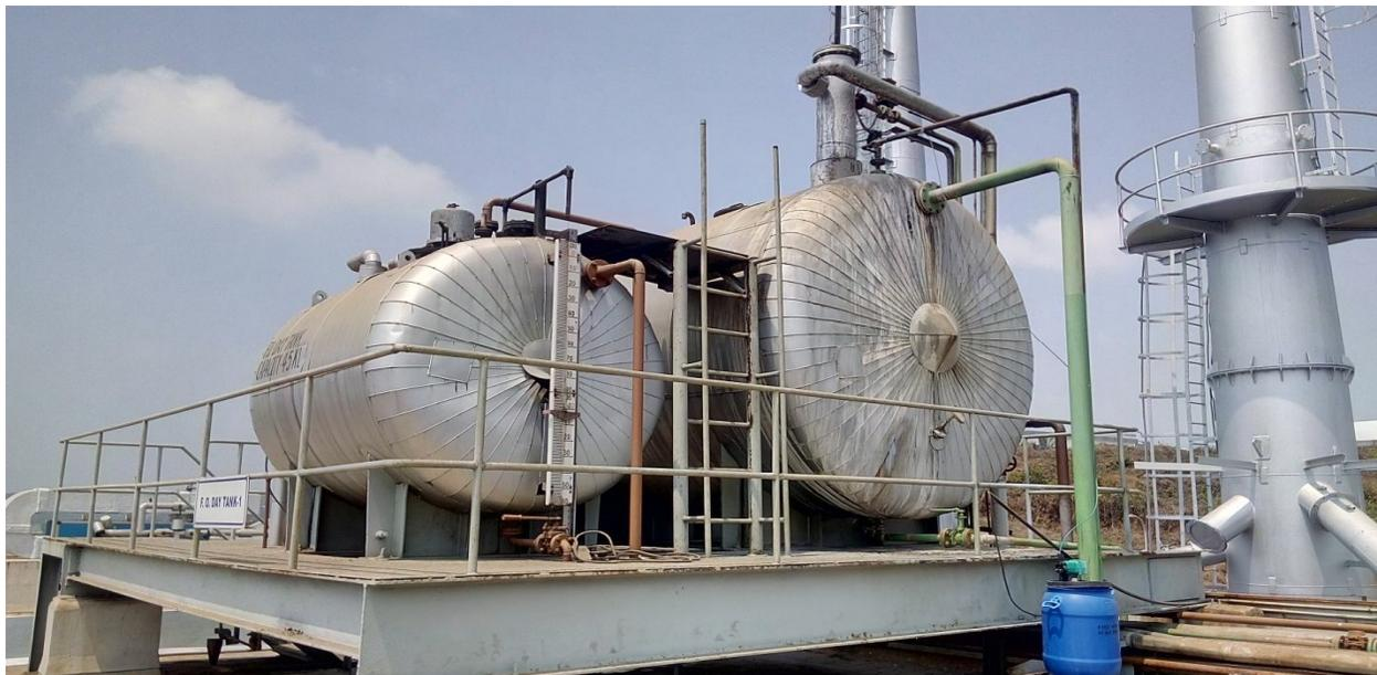
It is recommend to install new feed water tank of capacity 8 cu.mtr with steam purging system in it to heat feed water upto 85 – 100°C.and use existing tank as soft water storage tank.
